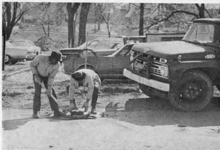
The unexpected arrival of an early spring in whimsical Missouri has lent itself to campus beautification. Here two maintenance workers fill potholes caused by the severe freezing weather over December and January. photo by Bill Leslie
